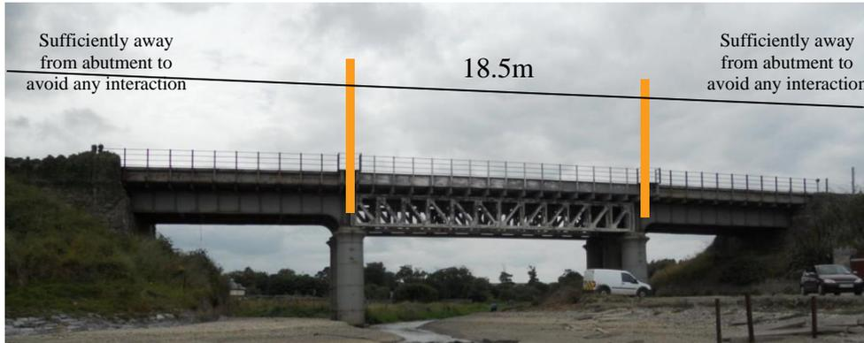
**Figure 6-9: Proposed OHLE frame location – arrangement 2 (source: Iarnród Éireann)**
