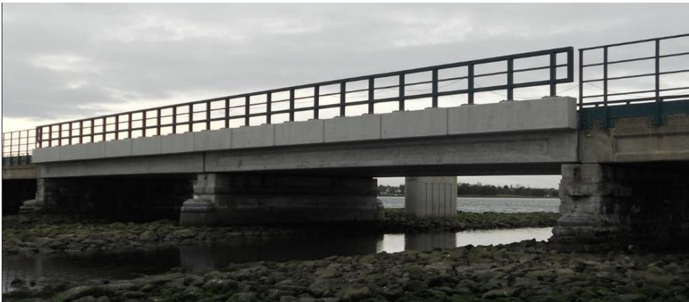
**Figure 3-5: UBB30 replaced spans (4 and 5) and reconstructed Pier 4 (source: Iarnród Éireann)**
