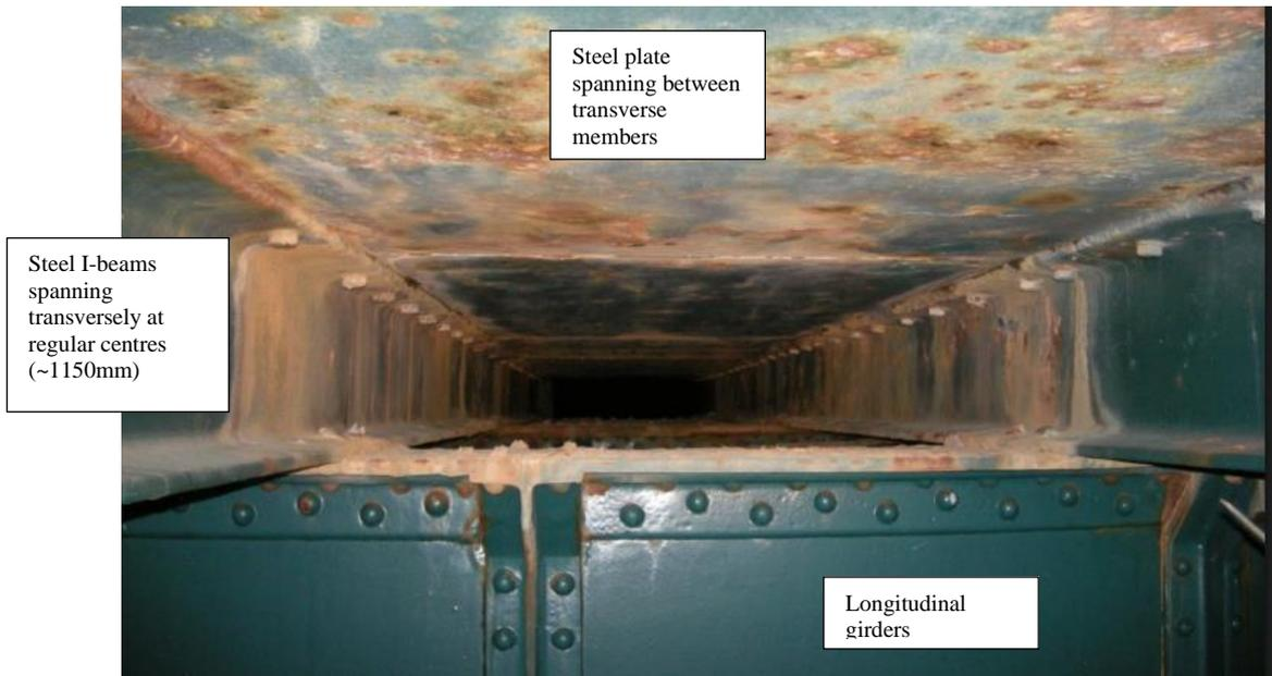
**Figure 7-3: UBB72 deck steelwork arrangement (source: Iarnród Éireann)**
