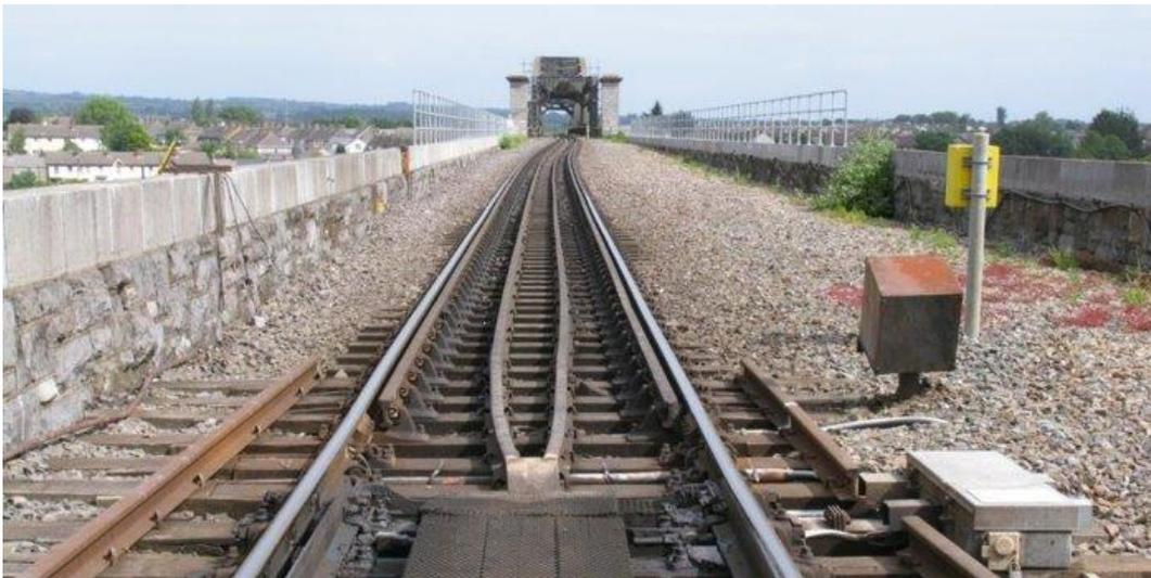
**Figure 8-6: UBB82 View of deck arrangement (source: Iarnród Éireann)**
