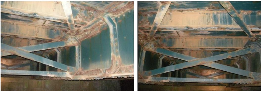
Figure 7-7: Intermediate pier diaphragm with plan bracing (source: Iarnród Éireann)
